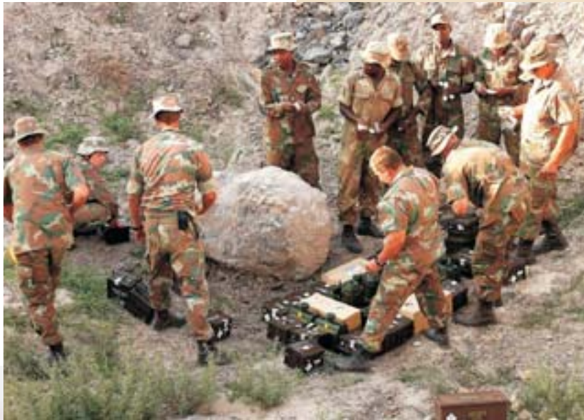
Members of 2 Field Engineer Regiment prepare to demolish a crater.
